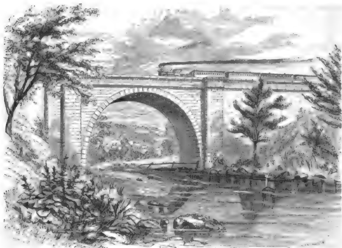
Viaduct of the Cheshire Railroad at South Keene.
